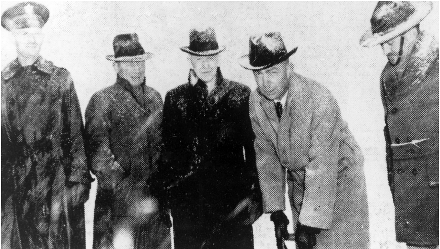
Groundbreaking for Hill Field, 12 January 1940. Left to right: Maj I.A. Luke, Ordnance Depot commander; Herbert A. Snow, Salt Lake City Chamber of Commerce president; Utah Governor Henry H. Blood; Frank Browning, and Capt K.I. Hastings, constructing quartermaster.
