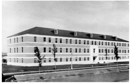
Barracks and Post Exchange, Hill Field, 1941.
