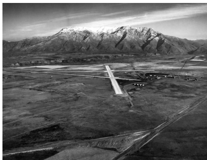
Ogden Air Depot, Hill Field, November 1940. Depot construction is visible at right; Weber Canyon is visible at top right.
