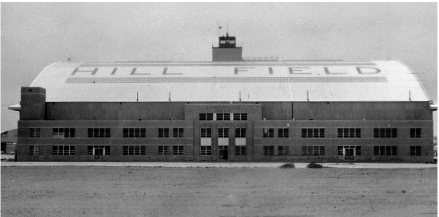
Transient Aircraft Operations and Maintenance Hangar, Hill Field, 1941.
